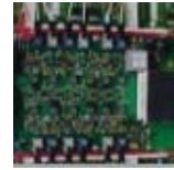
Auxiliary Power Supply
