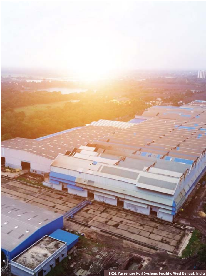
TRSL Passenger Rail Systems Facility, West Bengal, India
